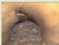
Drainage Pipe Collapse Under Stress (Courtesy Maverick Inspection Ltd)
