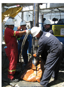
Cable being clamped to casing/production tubing
