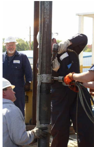
Cable being clamped to casing/production tubing
