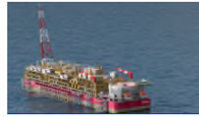
Akpo All Electrical FPSO
