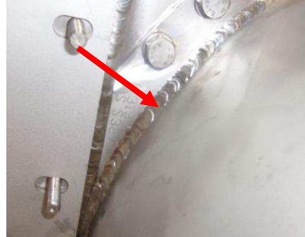
Weld properly filled and cleaned
