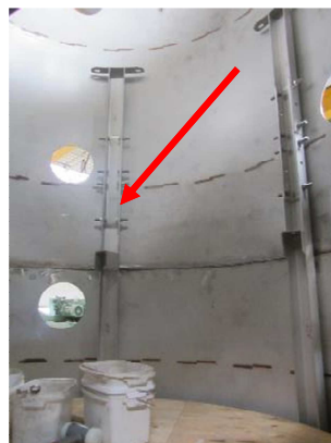
Installation of Support structures vertical vessel
