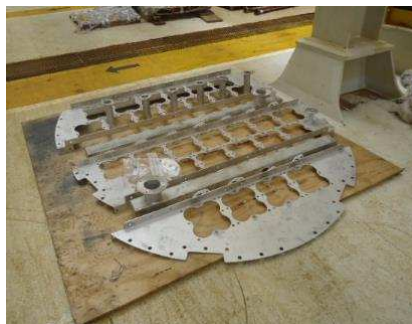
Spiraflo deck positioned – ready to be installed in the vessel
