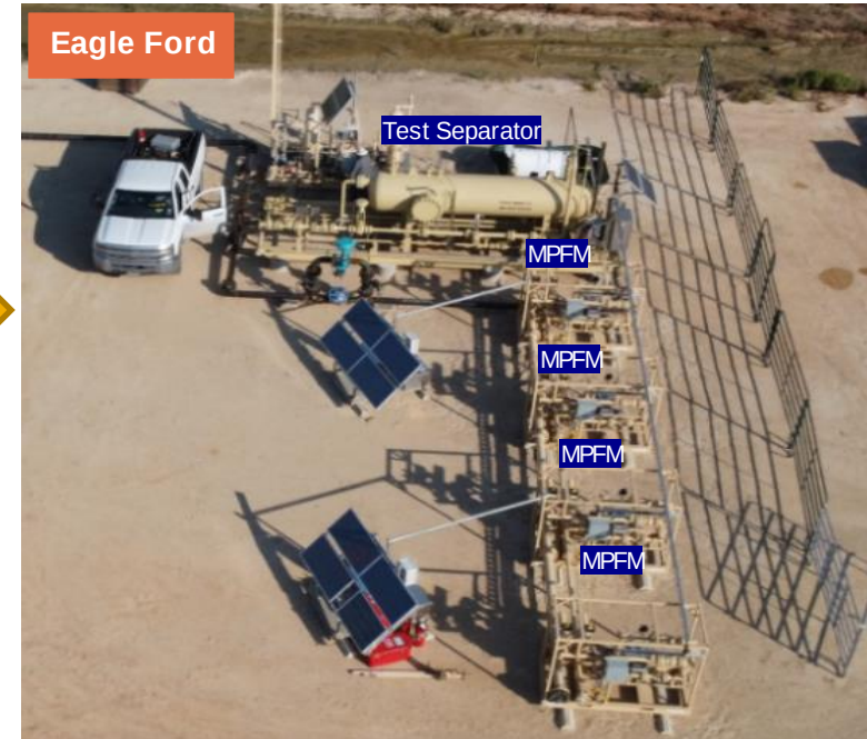
Hybrid 4 well pad combining MPFM and only 1 test separator
