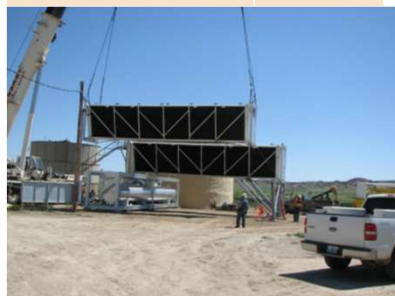
Installation of the energy converter. The unit was installed and commissioned in four weeks
