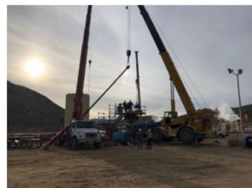
Installation of Insulated Tubing
