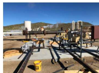
Equipment Pad and Partial Installation
