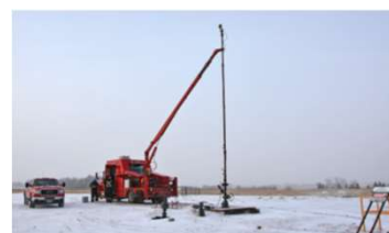
Slickline unit with temperature probe set up over the abandoned well
